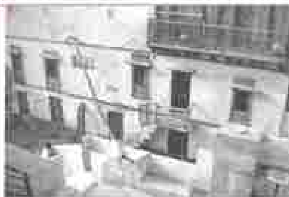
Rooftop harvesting was common across the towns and villages of the Thar. Rainwater that falls on the sloping roofs of houses is taken through a pipe into an underground tank (circular holes in the ground), built in the main house or in the courtyard. The picture above shows water being from a neighbour's roof through a long pipe. Here the neighbour's rooftop has been used for collection of rainwater. The picture shows a hole through which rainwater flows down into an underground tank.
